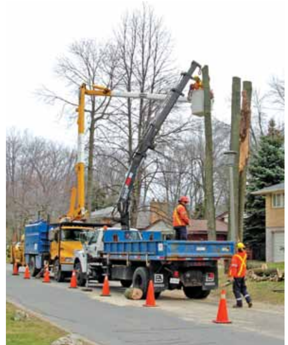
Aerial device and crane
