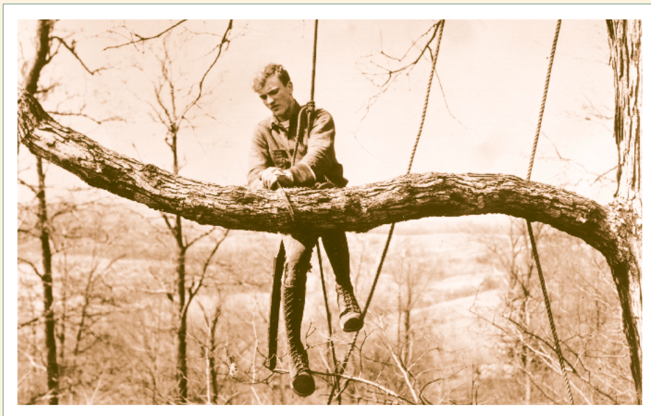
Following World War II, the well-dressed tree surgeon wore surplus military britches and high-lacing boots. Climbers used manila ropes, and a bowline on a bight served as a saddle until bosun's seat and barrel stave saddles were introduced.
